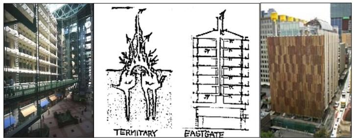
Figure 6: Eastgate Building in Harare, Zimbabwe and CH2 Building in Melbourne, Australia
