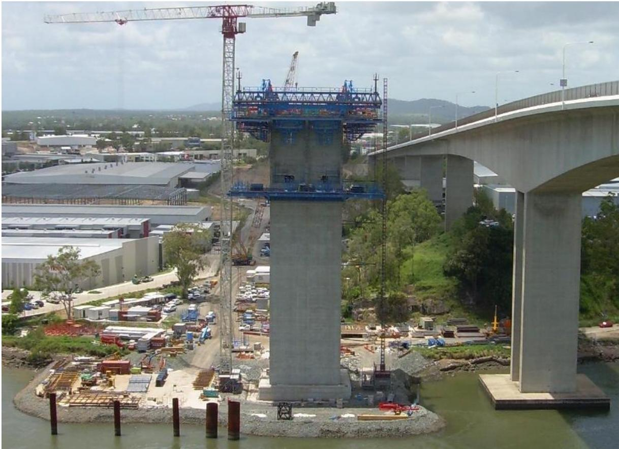
**Figure 7 – View of Pier 6 Showing Construction Platform (Future Ship Arrestor), Pile Cap and Column with Pier Head Complete, Ready for Balanced Cantilevering**
