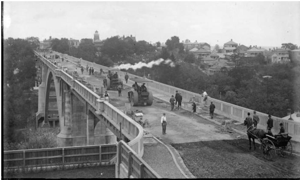
Figure 2 – Steamrollers load testing Grafton Bridge prior to opening in 1910
