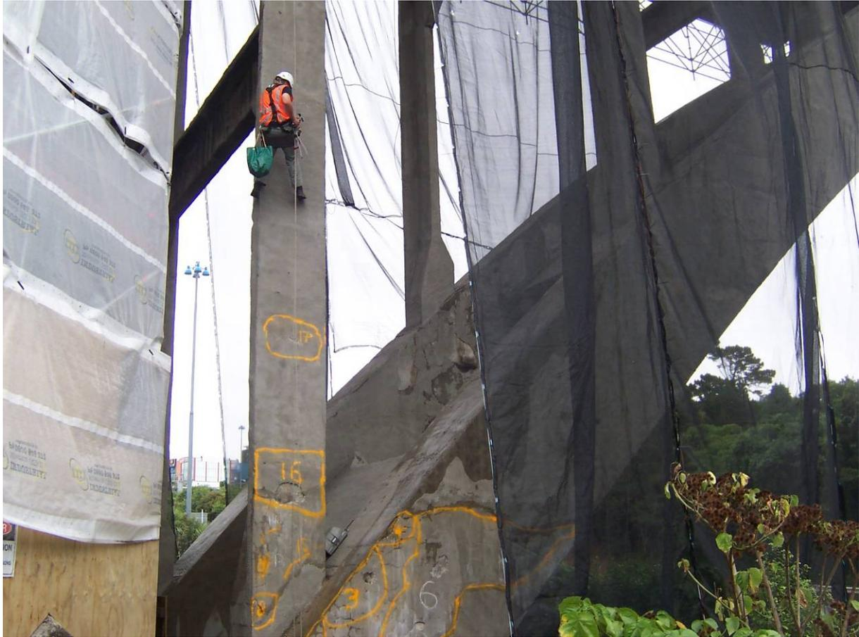
Figure 11 – High Level Inspection by Rope Access
