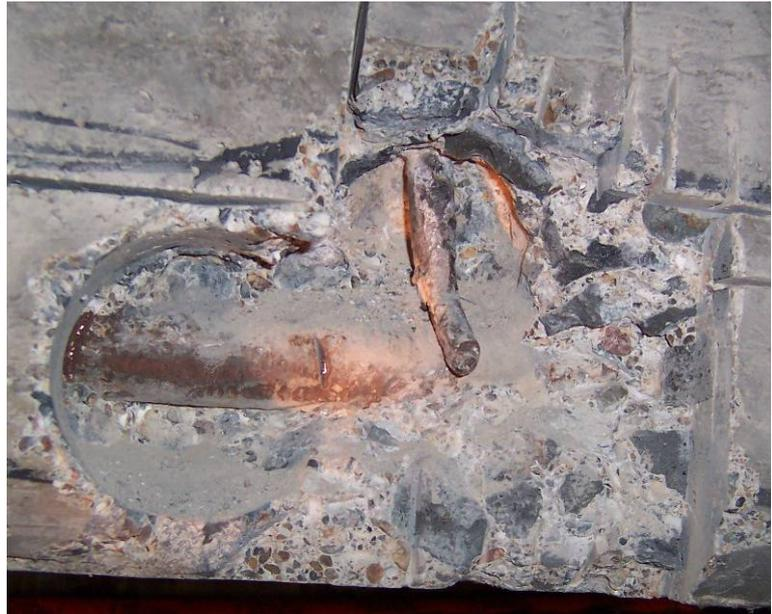
Figure 6 – Shear Bar Photo showing exposed reinforcement
